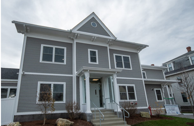
323 MANCHESTER STREET 22 UNITS MANCHESTER Supportive Housing
