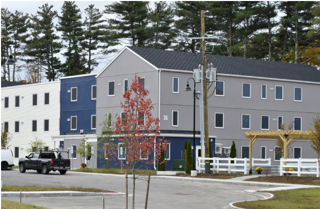
RIVER TURN WOODS 40 UNITS CONWAY General Occupancy
