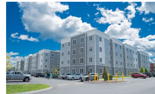
Monahan Manor Apartments in Nashua, NH
