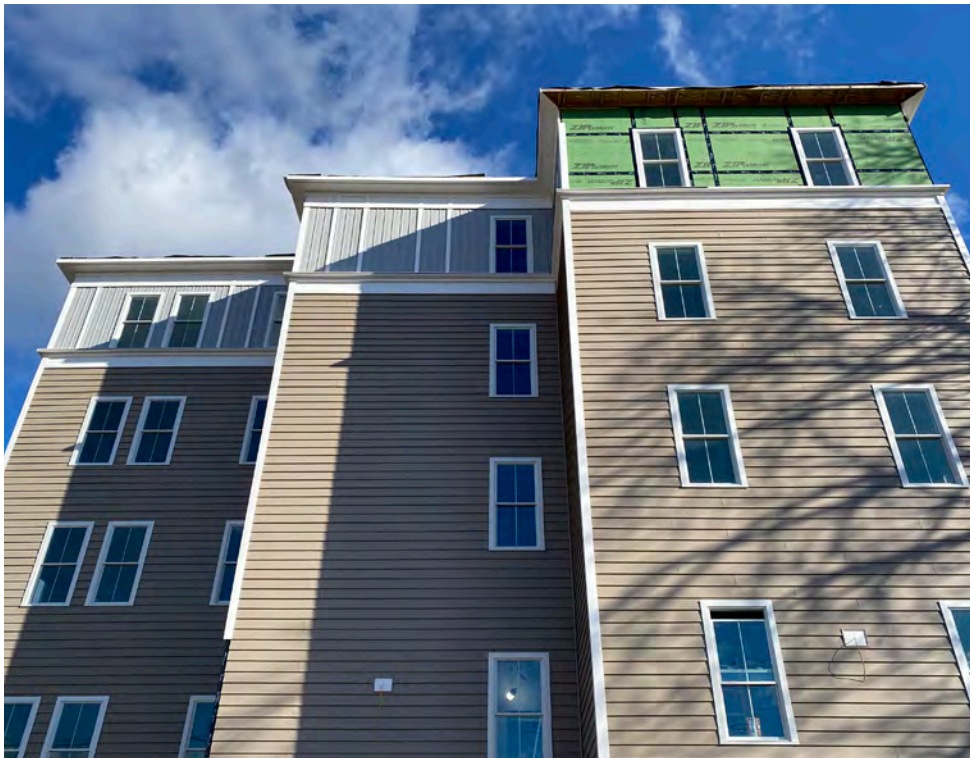
The Salinger development during construction. Photo from the City of Rochester.
