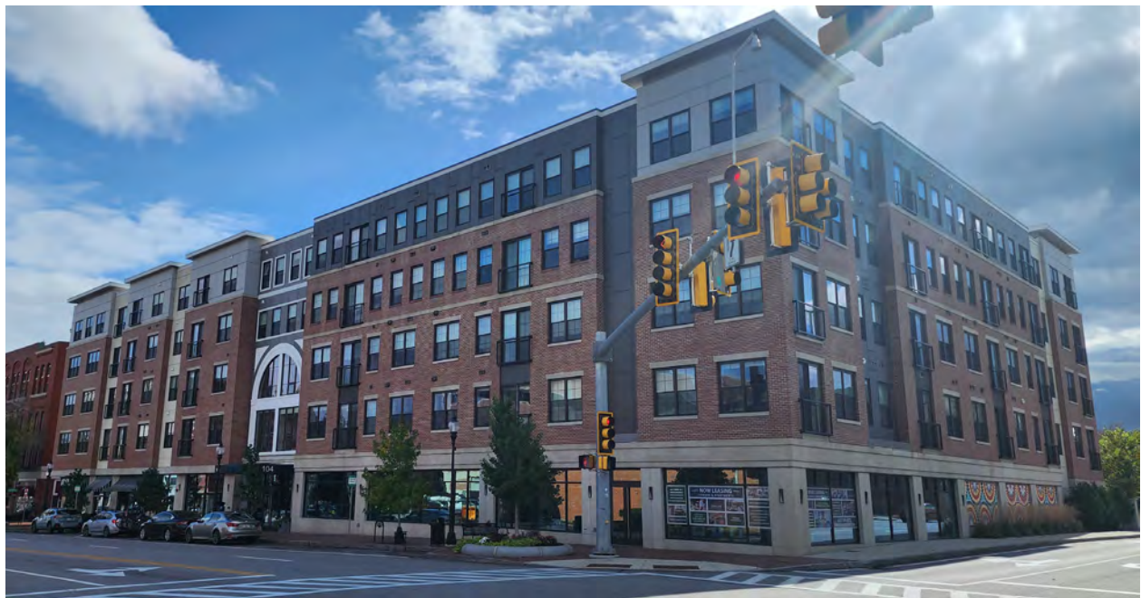
View of the Orpheum Apartments. Photo from the City of Dover.
